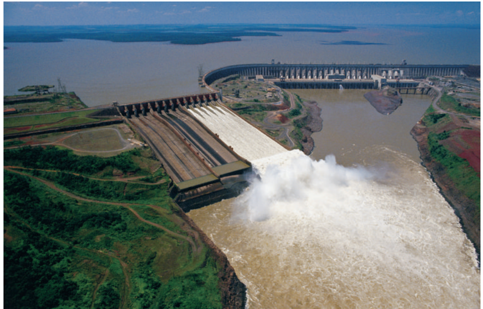
FIGURE 4.14 | ITAIPÚ DAM The largest dam in Latin America, the Itaipú blocks the flow of the Paraná River on the border between Paraguay and Brazil. The power station at Itaipú generates all of Paraguay's electricity needs and much of southern Brazil's power. (Sue Cunningham/Worldwide Picture Library/Alamy.com)
