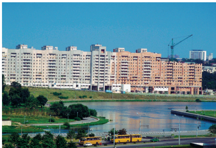
FIGURE 9.16 | MINSK This row of mass-produced apartment houses is found along the banks of the Svisloch River in Minsk, Belarus. (Nik Wheeler/Corbis/Bettmann)
