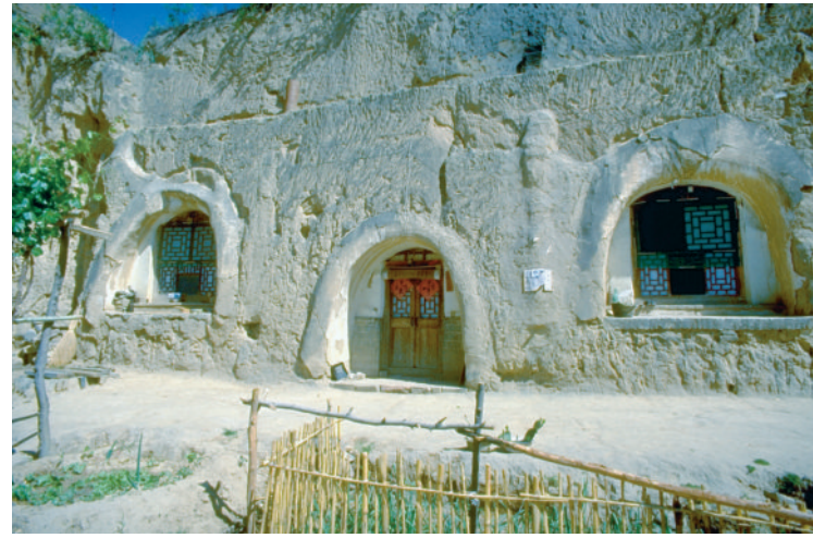
FIGURE 11.15 | LOESS SETTLEMENT This photo shows a typical subterranean dwelling carved out of the soft loess sediment in central China. This area is prone to major earthquakes that take a high toll on the local population because of dwelling collapse. (Christopher Liu/ChinaStock Photo Library)
