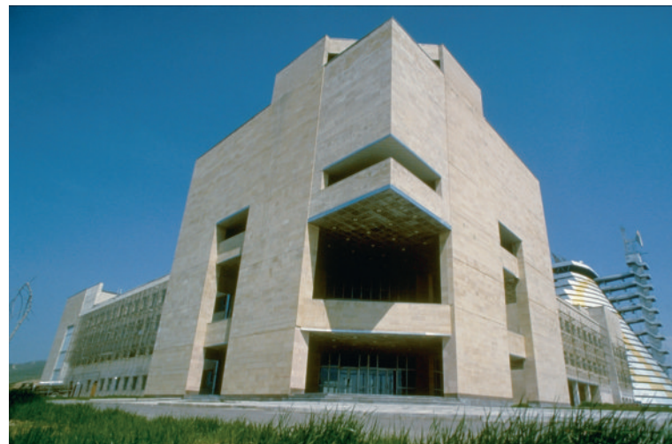
FIGURE 10.30 | TARKENT HELIOSTATION IN TASHKENT, UZBEKISTAN Despite its generally poor economic statistics, Uzbekistan boasts a relatively well-developed medical, educational, and technological infrastructure. The Tarkent heliostation focuses the sun’s rays to generate the extraordinarily high temperatures needed to produce super-pure industrial minerals. (Novosti/Getty Images, Inc.—Liaison)
