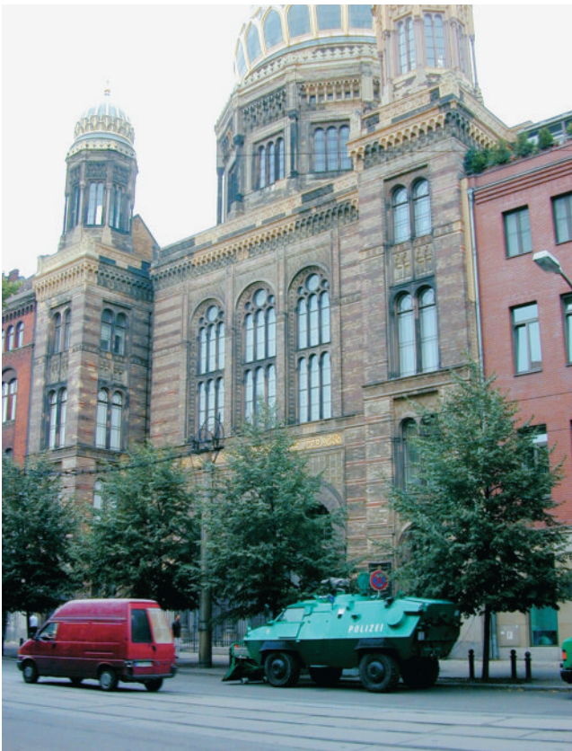
FIGURE 8.24 | JEWISH SYNAGOGUE IN BERLIN Before World War II, Berlin had a large and thriving Jewish population, as attested to by this synagogue built in 1866. However, during the Nazi period, the Jewish population was forcibly removed and largely exterminated. This synagogue was then used by the Nazis to store military clothing until it was heavily damaged by bombing. After the war, it was restored and opened again in 1995 as both a synagogue and a museum. ( Les Rowntree )
