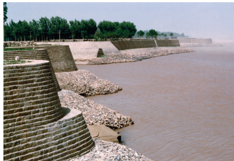
FIGURE 11.4 | FLOODING ON THE NORTH CHINA PLAIN Major floods on the Huang He River have occurred throughout history, sometimes inundating large sections of the North China Plain. At other times, severe droughts affect the same region. Extensive dikes have been built along much of the river to protect the countryside from flooding, as seen in this photo taken near the historical city of Kaifeng. (Yang Xiuyun/ChinaStock Photo Library)
