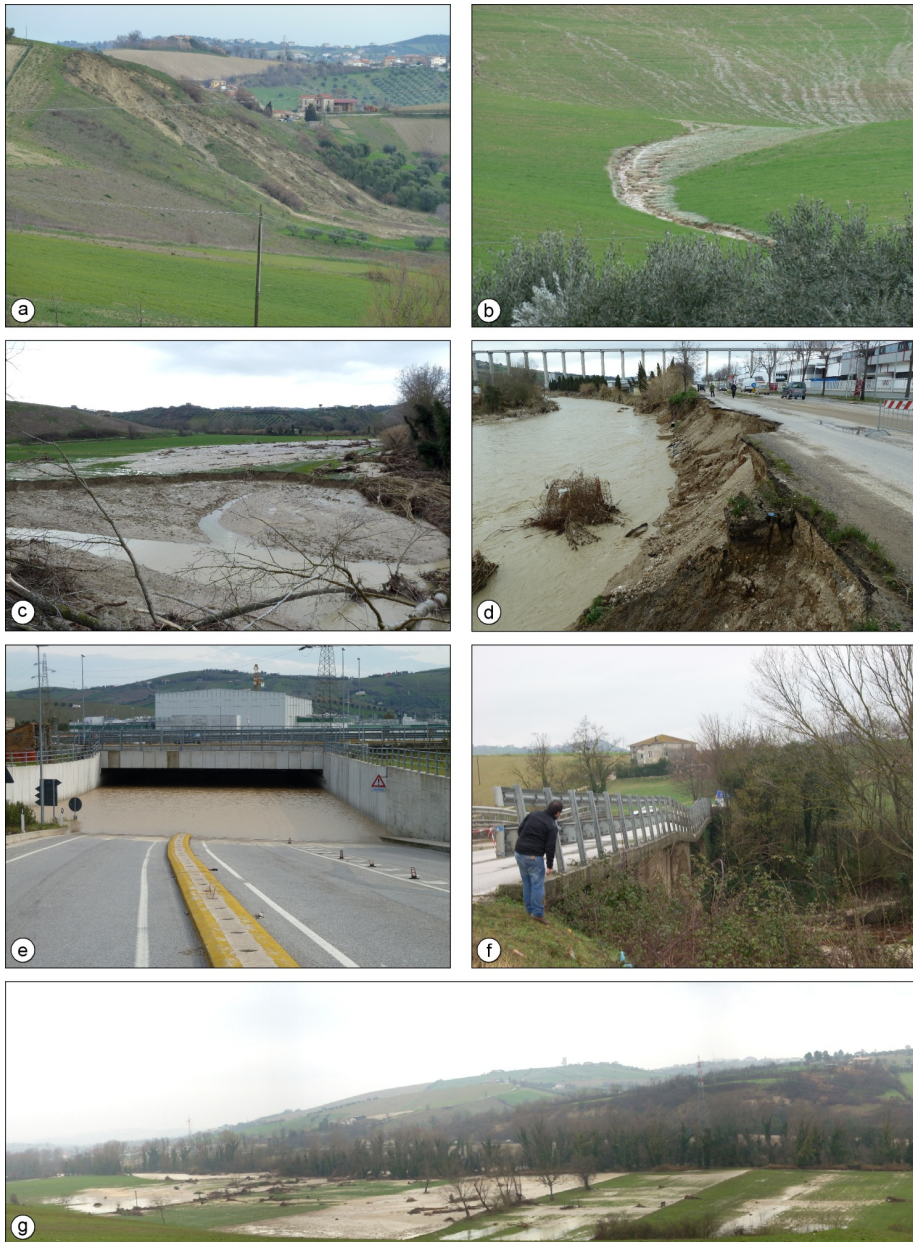
Fig. 10. Landform triggered by the 2011 heavy rainfall event: a) Mosciano S. Angelo, rapid earthflows; b) Pineto, gullies on the coastal slope; c) F. Salinello, crevasse splay and fluvial erosion scars; d) F. Salinello, fluvial erosion scarp affecting the valley road; e) F. Vomano, main river flooding affecting main roads; f) F. Salinello, damage to a bridge; g) F. Salinello, flooding and crevasse splays along the main alluvial plain.
