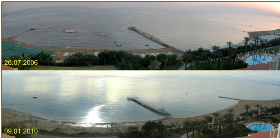
Fig. 12. Two panoramic views of the Perissia Hotel Beach at 26.07.2006 and 09.01.2010 showing the before and after remedial measures
