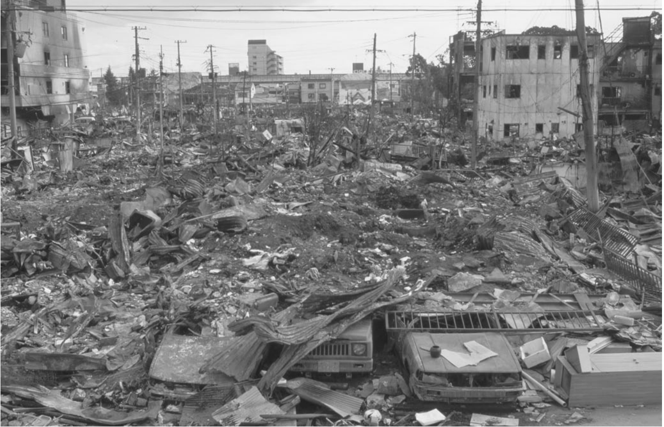
FIGURE 8.35 Damage from the Kobe earthquake in 1995 (Japan).
