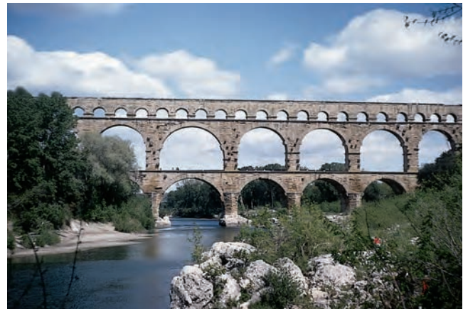
Figure 9.14 Nîmes, France. Aqueducts outside of Nîmes, France were built during the Roman Empire, about 2000 years ago. © Alexander B. Murphy.
