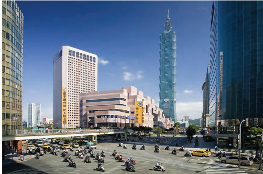
Figure 4.21 Taipei City, Taiwan. The Taipei 101 Building, the World's tallest building. ©José Fuste Raga /Age Fotostock America, Inc.
