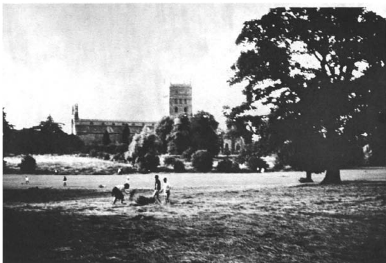
Fig. 66 The medieval English vineyard site at Tewkesbury, Gloucestershire. The ground slopes gently northwards to a ditch in the middle ground of the picture. Surely a frost hollow site, which suggests that the medieval cultivators were not much troubled with late frosts in May after blossom time.
